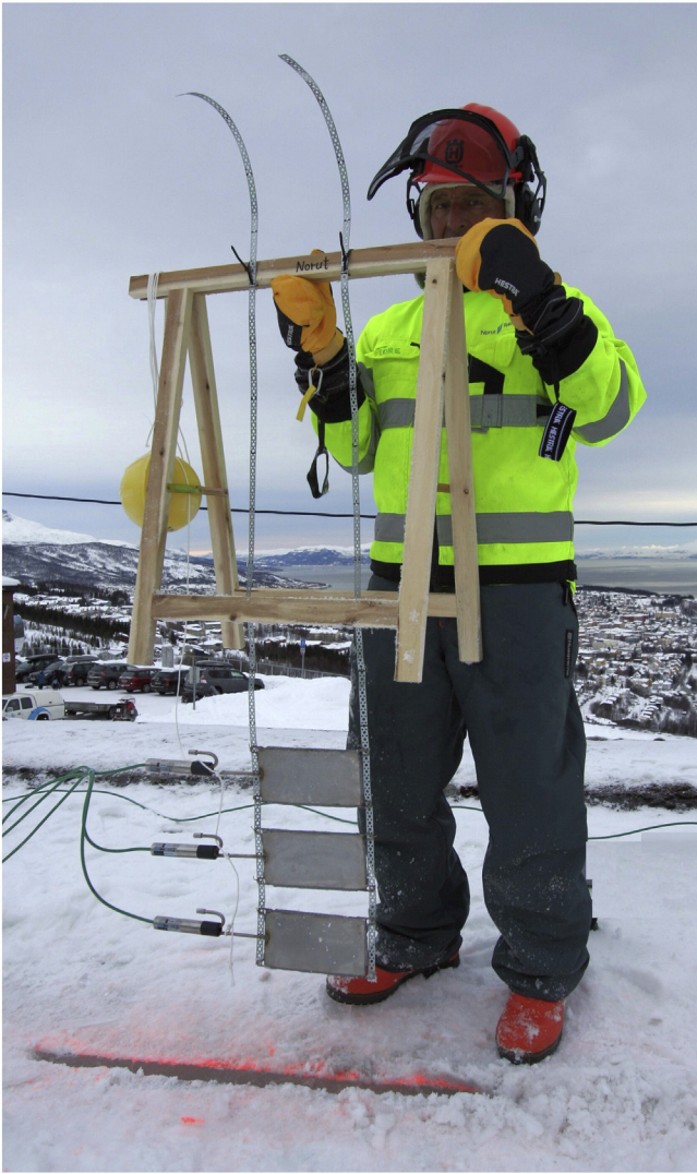
Fig. 3. Installation of stress cells at Station 5 on 12 February 2013.
